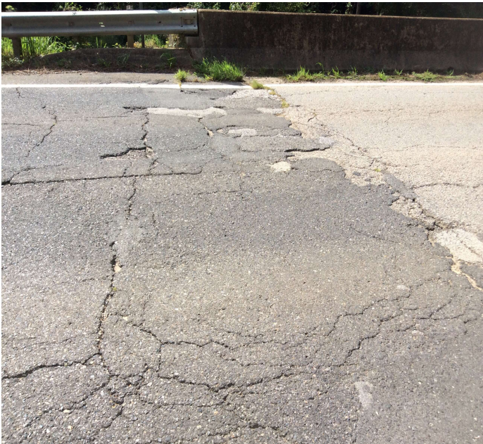
PHOTO 1 Description East end of bridge asphalt approach has settled.
